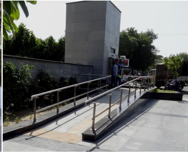
Figure 11-5: Lift access to subway crossing
