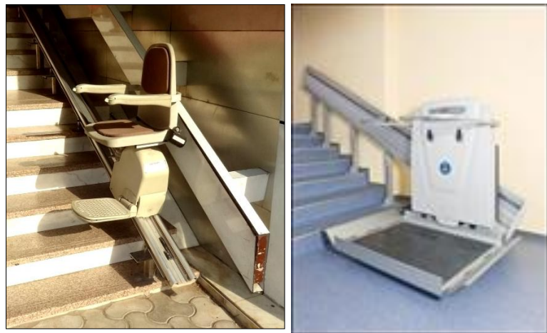
Figure 7-18: Platform chair lift and platform lift
