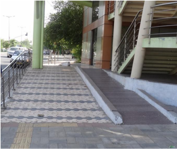
Figure 11-6: Lift access to Foot Over Bridge
