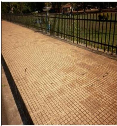
Figure 5-1: Chequered tile on footpath
